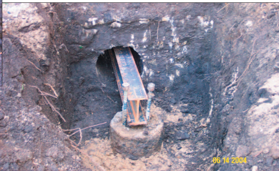
Underpinning of exterior foundation wall.
