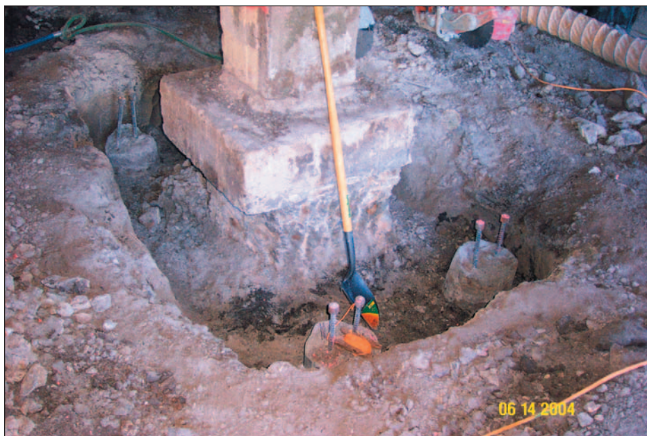
Underpinning of typical interior column footing.
